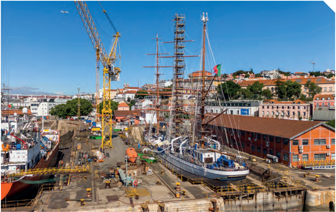
The three-masted barque NRP Sagres in drydock at Navalrocha
