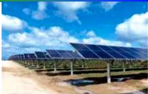
Location: China Capacity: 500MW Technology: SkyLine Tracking System + Bifacial Module (under construction)
